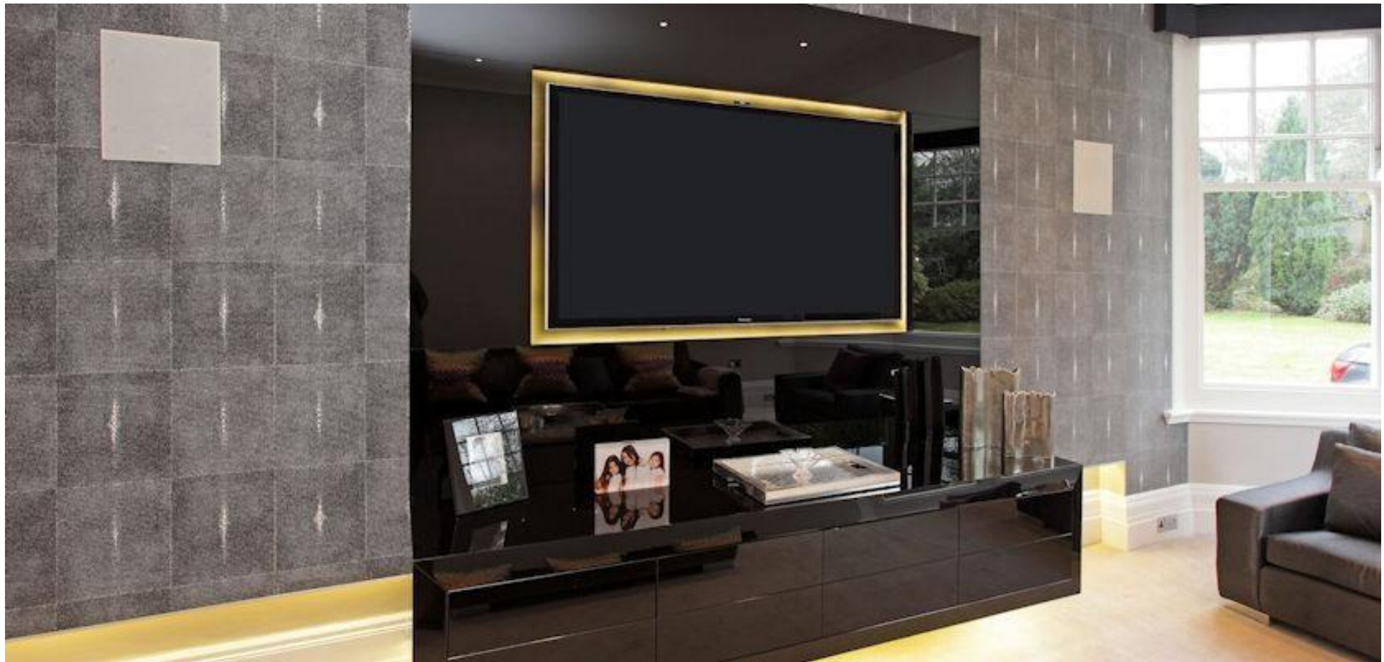
This wall-hung cabinet and television surround were clad in black glass. The doors are on push-to-open catches and the cabinet contains audio-visual equipment.
